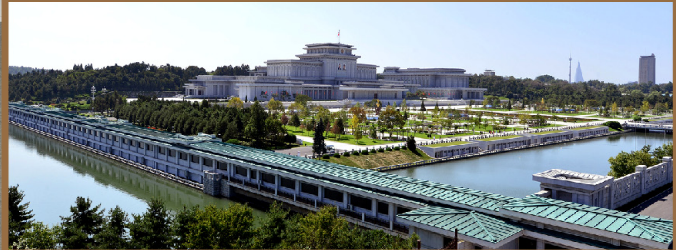
Travelator in the access corridor
