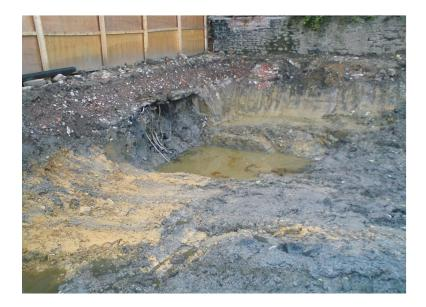
Figure 25.32: Soil contamination caused by underground storage tanks containing tar. (8)
