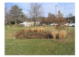
Figure 25.11: Intercepting nonpoint pollution between the source and waterway has been found to be successful. Pictured here, a bioretention cell, or rain garden, in the U.S, is designed to treat polluted storm water runoff from an adjacent parking lot. (4)
